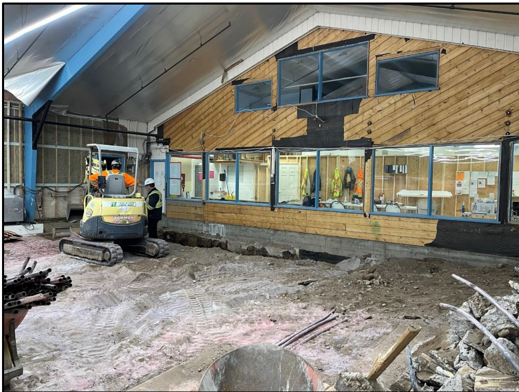
Construction works underway in the exciting upgrades to the curling club, skating rink and community hall complex
